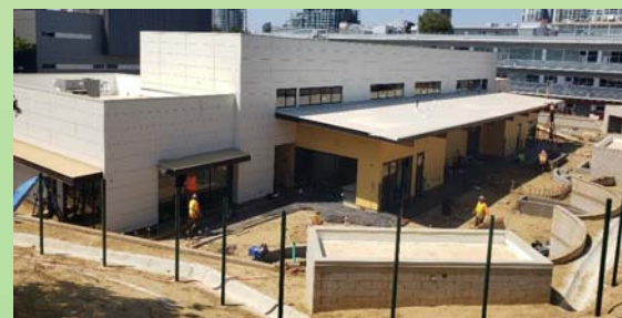
Construction – North Building
