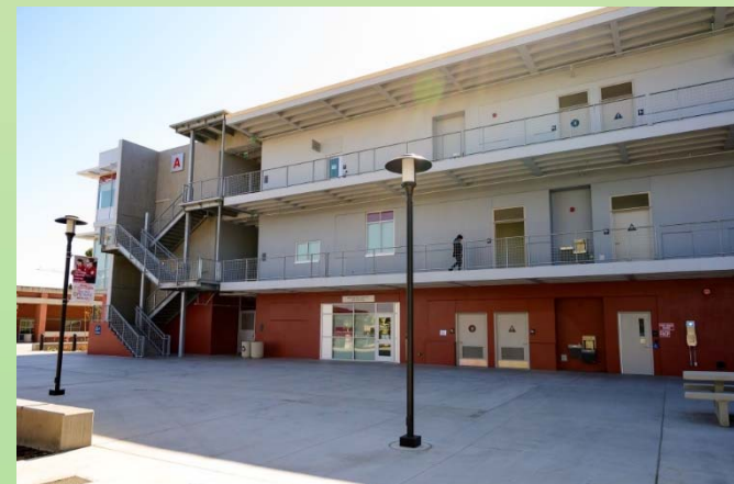
Engineering & Technology (“T” Bldg.)
