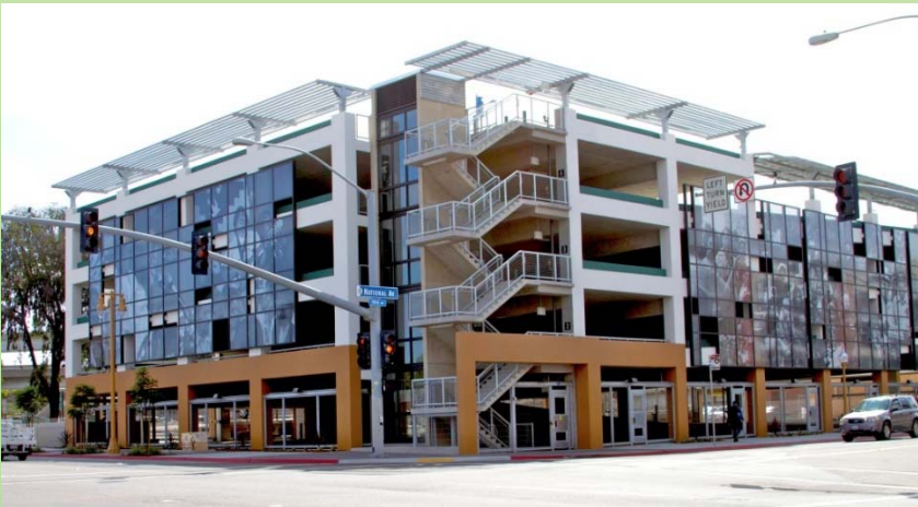
Cesar Chavez Parking Structure
