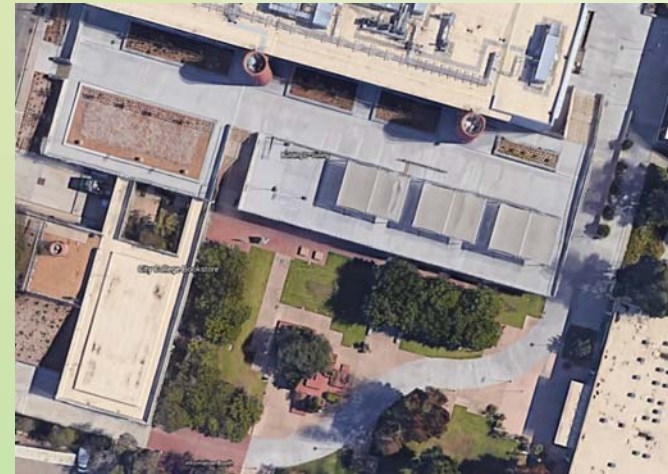
“D” Building roof courtyard
