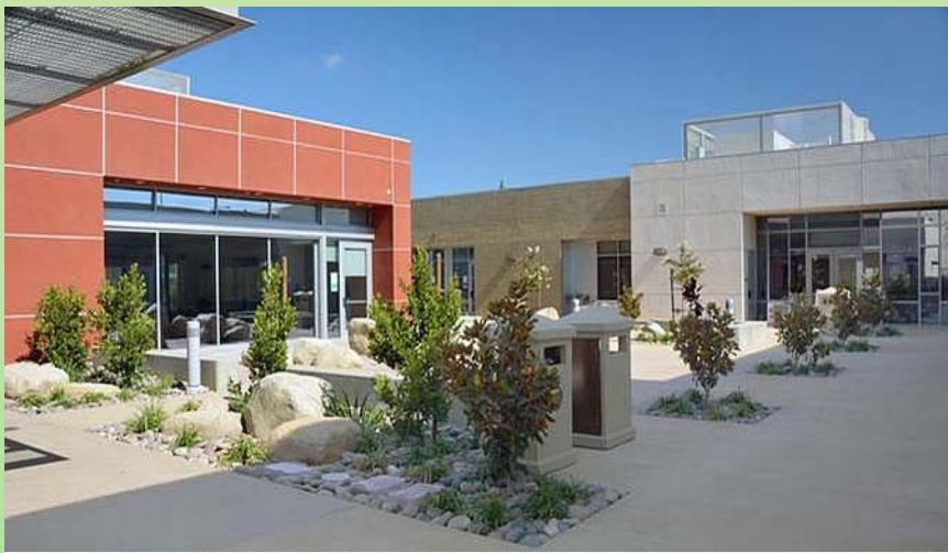
Fire Science/EMT Training Facility
