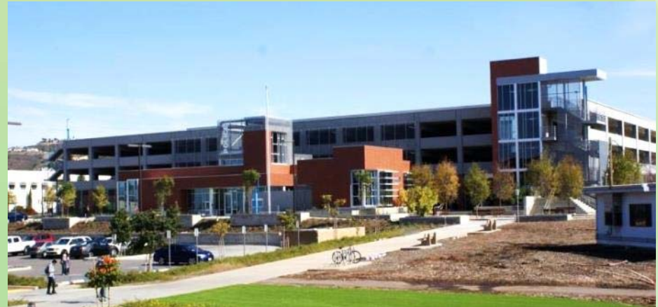
Police Station & Parking Structure
