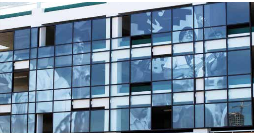
Photo murals depicting late labor leader César E. Chávez on the new parking structure in Barrio Logan.
