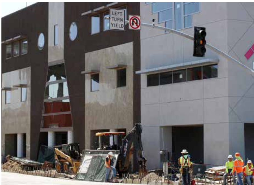
Construction workers are nearing completion of the César E. Chávez campus, set to officially open on October 28.
