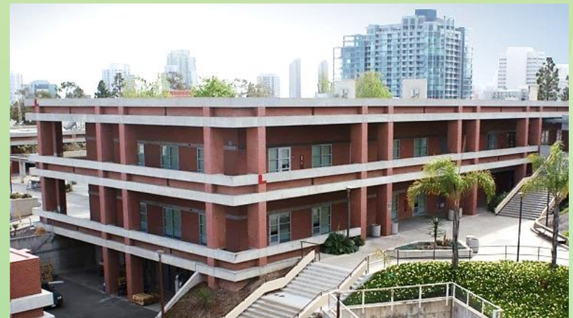
Academic Success Center ("L" Bldg.) Renovation
