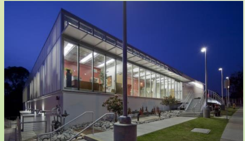
Health, Exercise Science and Athletics ("P" Building) Renovation
