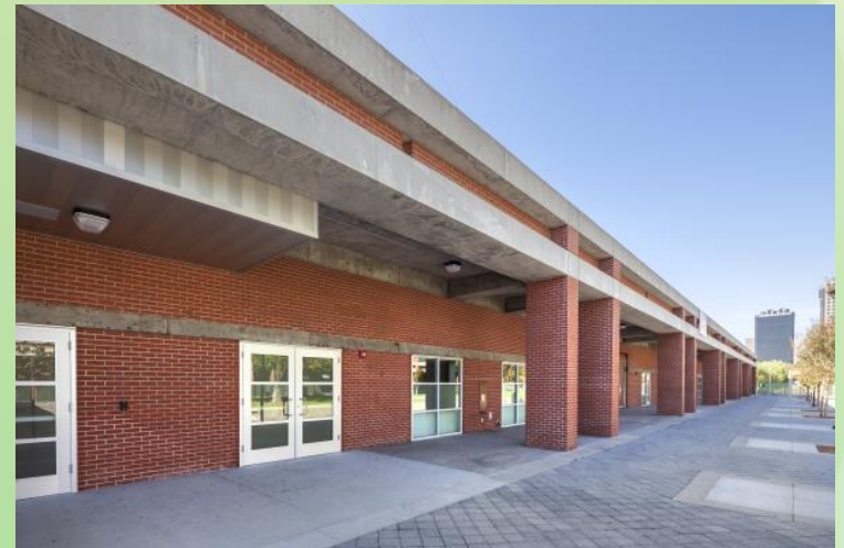
"C" Building Renovation
