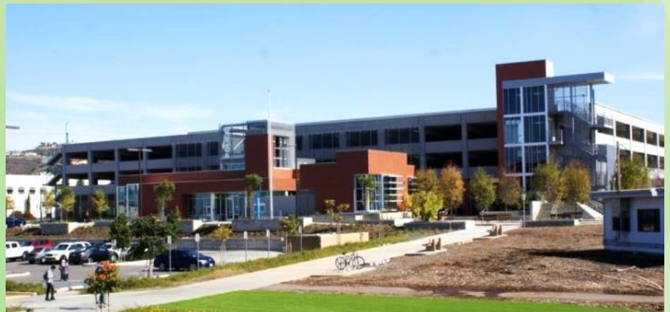
Police Station & Parking Structure
