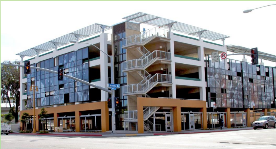
Cesar Chavez Parking Structure
